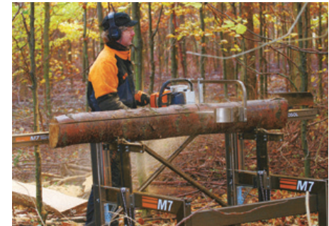
Svensson building the catwalk and platform with a mobile sawmill.
